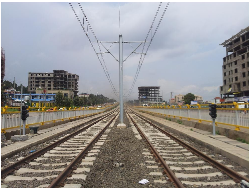
Figure 6: The nearly complete AA LRT System (photo taken on June, 2015)
