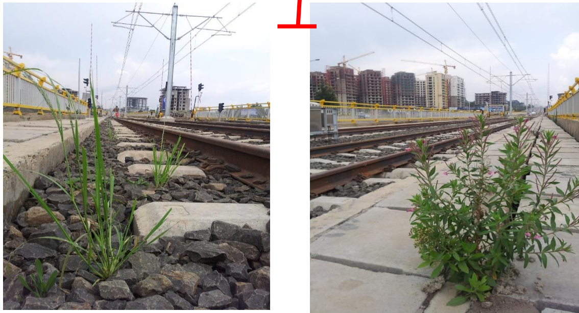
Figure 17: Plants got enough water and soil to grow on ballast around CMC roundabout
