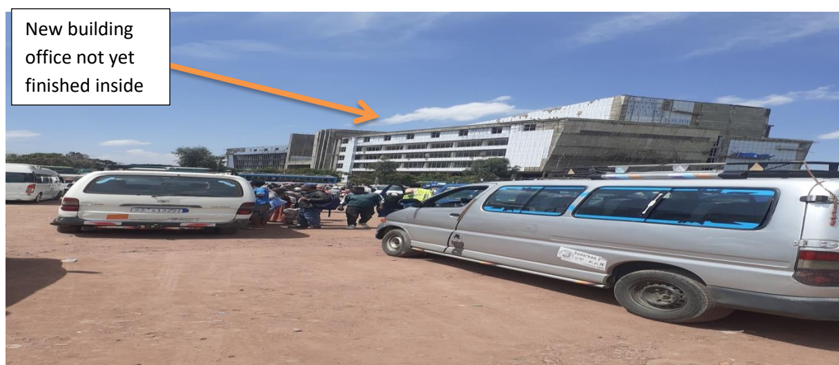
Figure 4.7: New building office not yet finished inside terminal kaloty terminal
