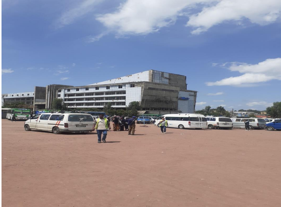
Figure 4.6 undergoing building construction in kality terminal
