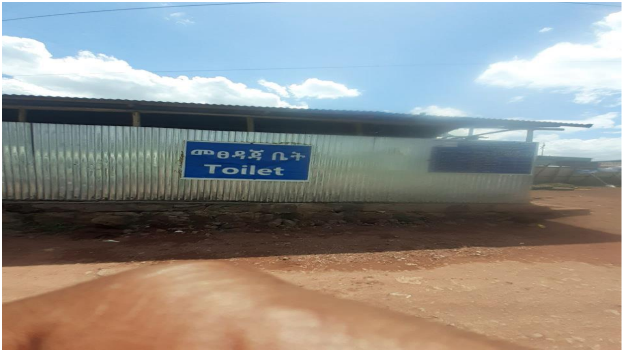
Figure D: Toilet area
