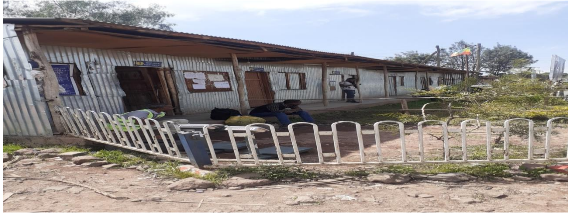
Figure 4.3 offices in kaliti terminal
