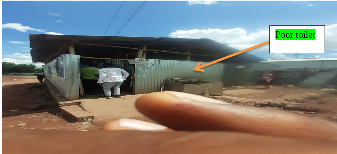
Figure E: poor toilet
