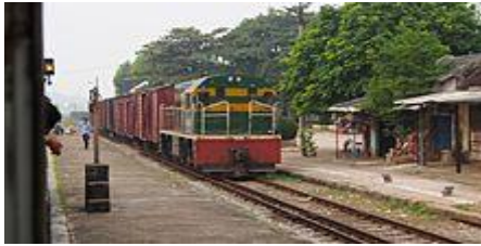
Figure 2.14: Dual gauge tracks at Đồng Đăng in Vietnam accommodates both meter gauge trains from Hanoi and standard gauge trains from Nanning and other cities in China.
