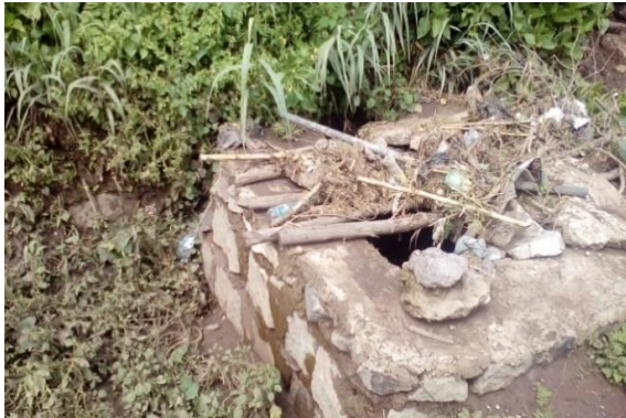
Figure 27 :The blocked sewerage needs machinery cleaner Akaki Kality Woreda 3.2018
