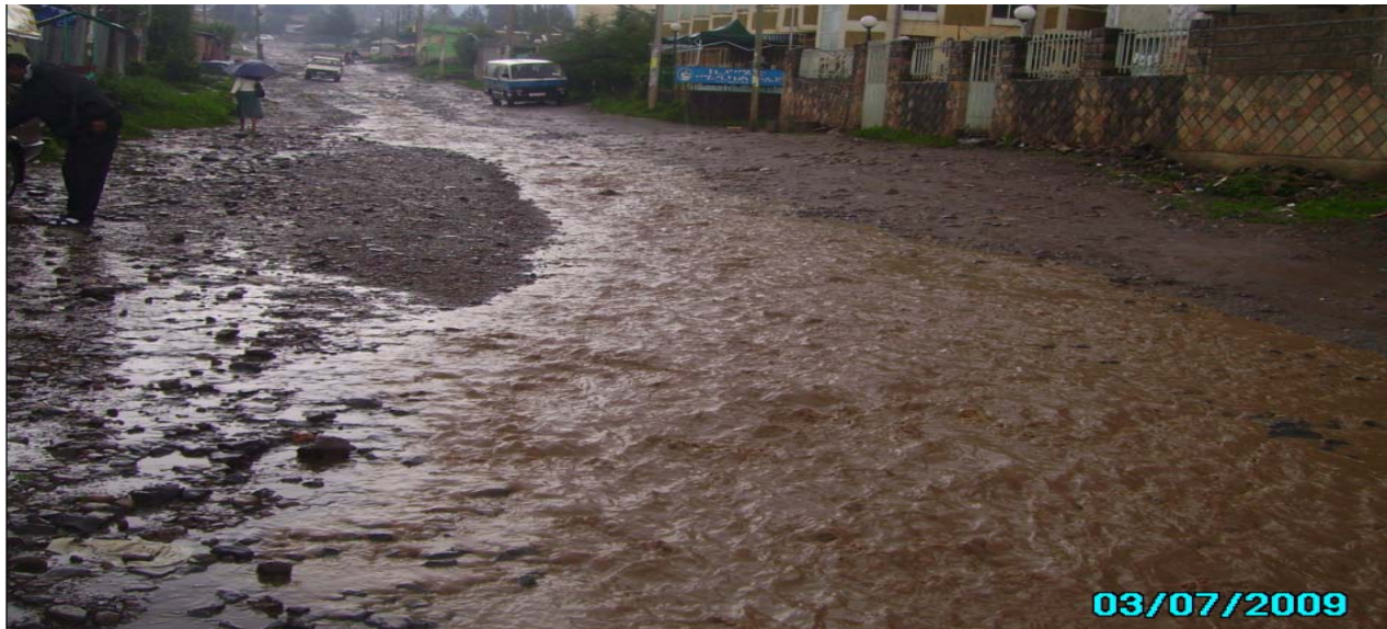
Fig-4.18 Flood over flowing on road surfaces kebele13/14 (source: Field survey, 2009).
