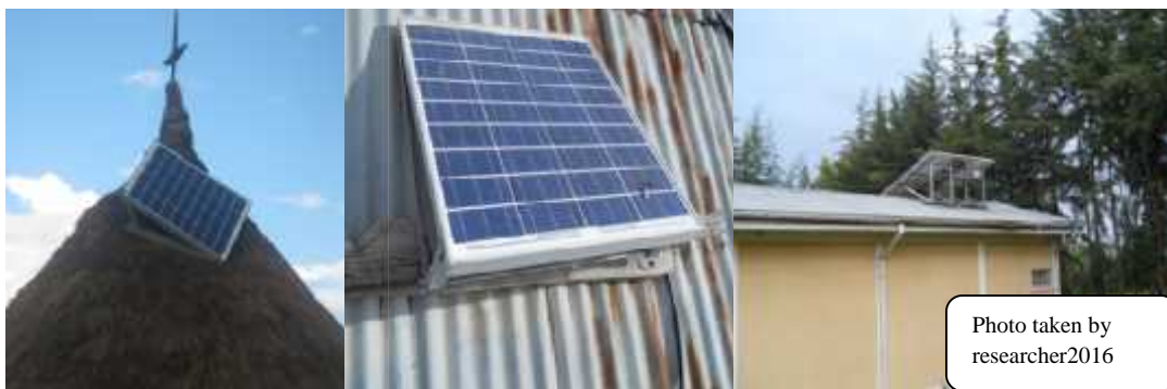
Figure 4.7 PV arrays should be oriented toward the solar window
