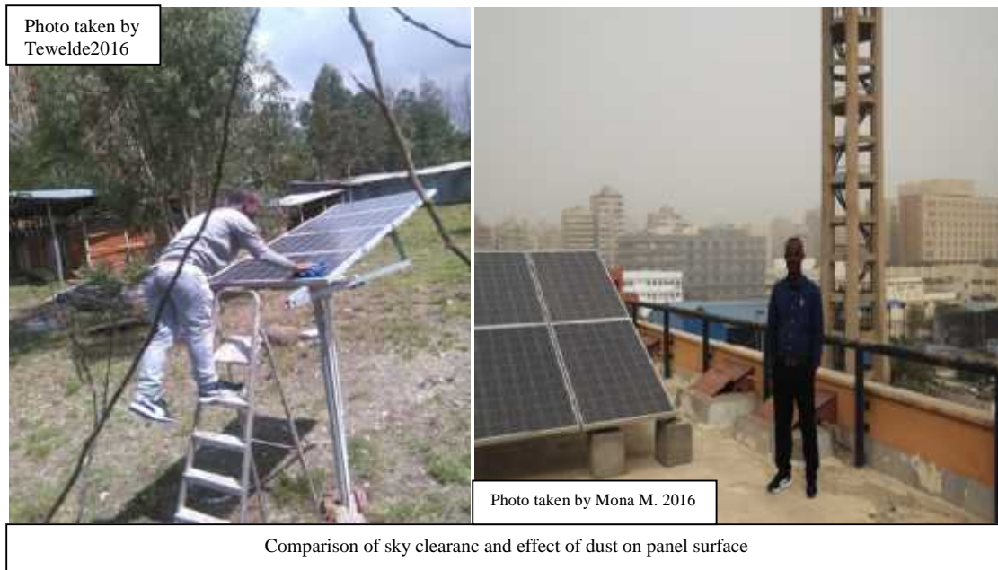
Figure 4.11 Photovoltaic panel must be kept clean
