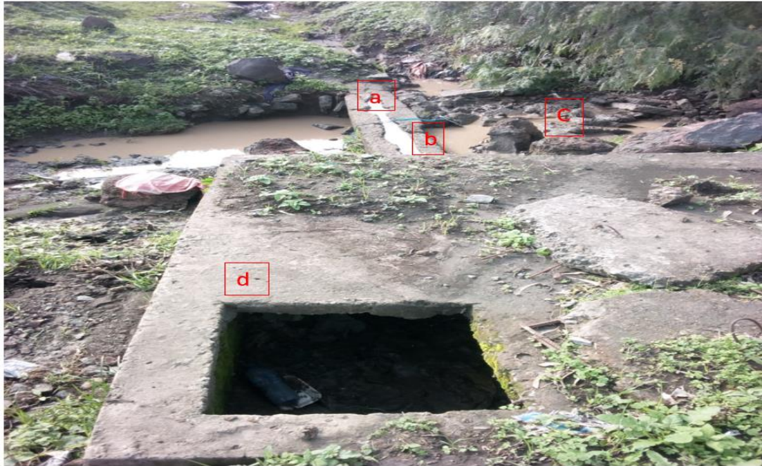
Figure 1-2 Faulty pipe alignment, and junction setting on flood route
