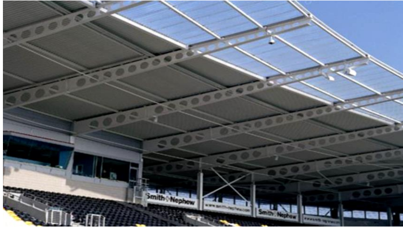
Figure 1. 1 Roof support beams(SAMEER S. FARES et al., 2016).
