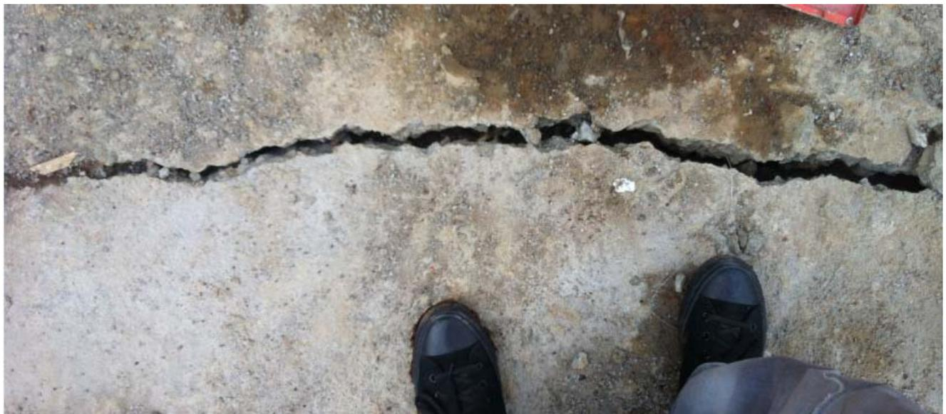
Fig. 25. Tunnel-1 Top Slab Waterproof covers Application and its crack [from source]
