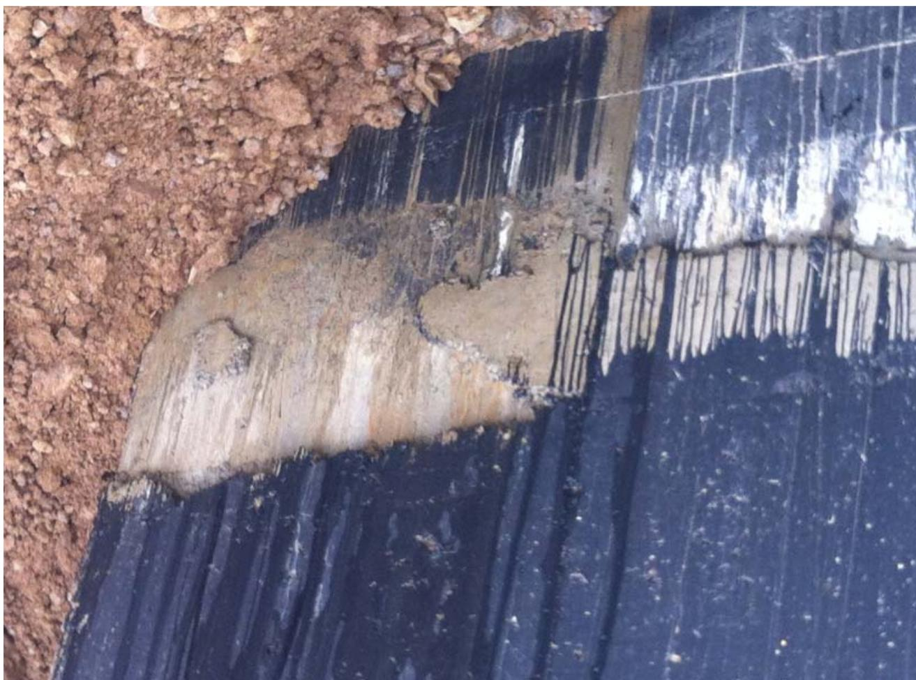
Fig. 24. Tunnel-1 Wall Waterproof Application and its Cover [from source]
