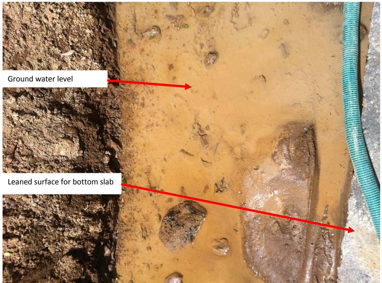
Fig. 23 Ground water level seen on bottom of Tunnel-1 cut level [from source]
