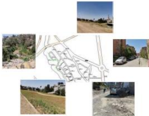
Figure 4.6: - Site images of Basha Wolde renewal project
