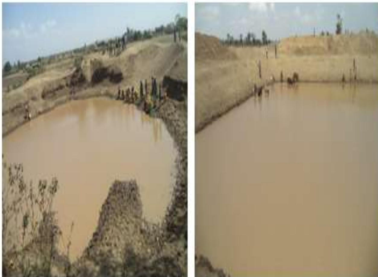
Figure.4.12. Photo shows pond water harvested from rainfall for consumption in the Bidara Faka Kebele.
