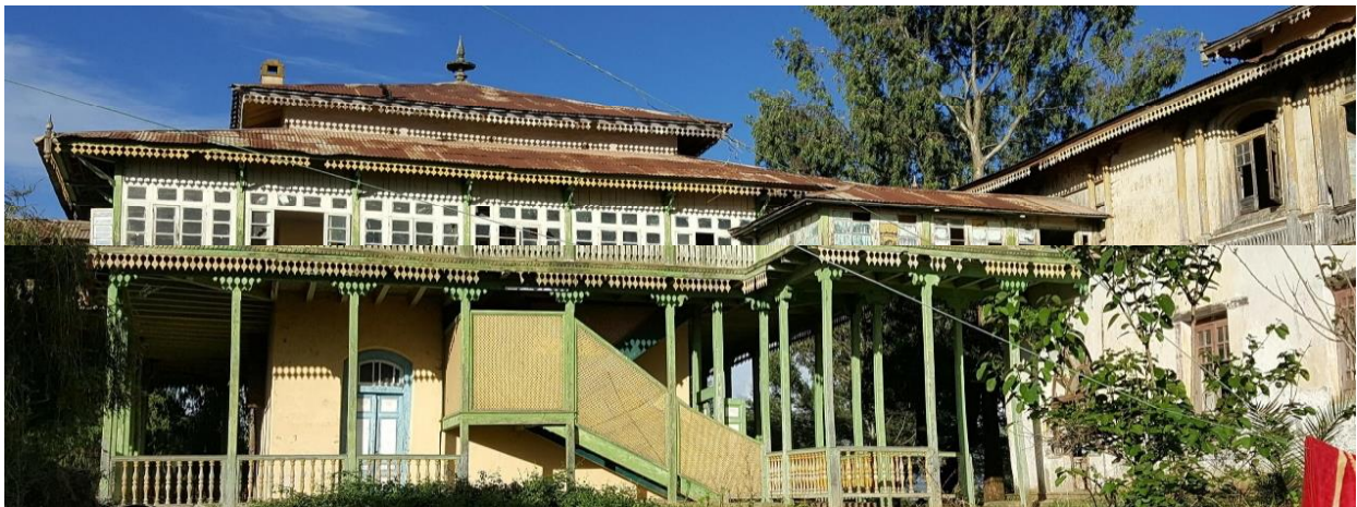
Figure: 3.5: Holata palace. The view of Block A and B with connecting bridge. Photo: By Researcher.
