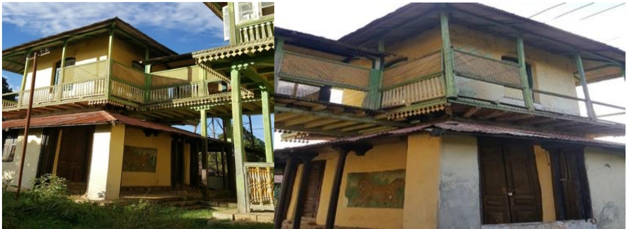
Figure 3.6- Block C North East Side View and Block C North West side view from left to right Photo: by Researcher
