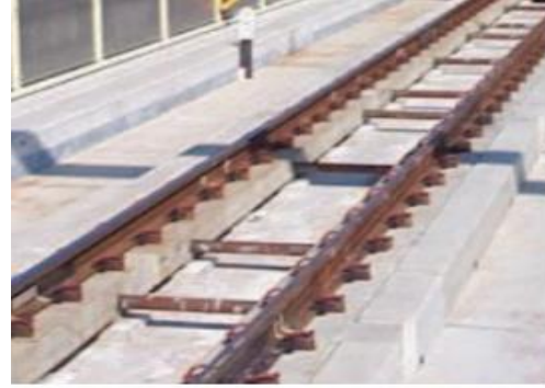
c) longitudinal concrete sleeper
