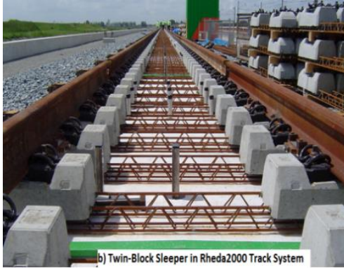
Figure 7: Types of Concrete Sleepers
