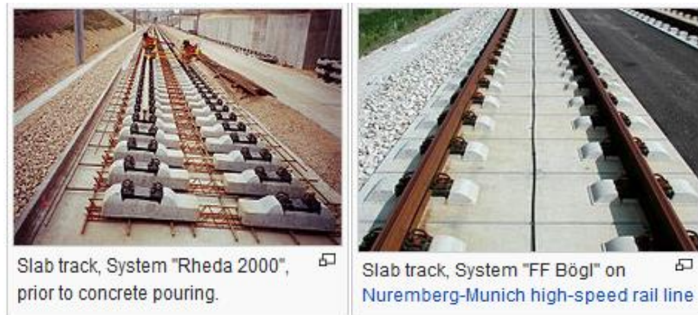
Figure 2: Rheda2000 Track system before and after monolithic in-situ cast
