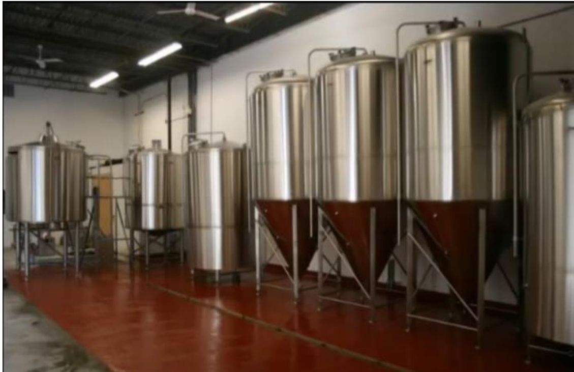
Figure 1.11 Brewery tanks welding
