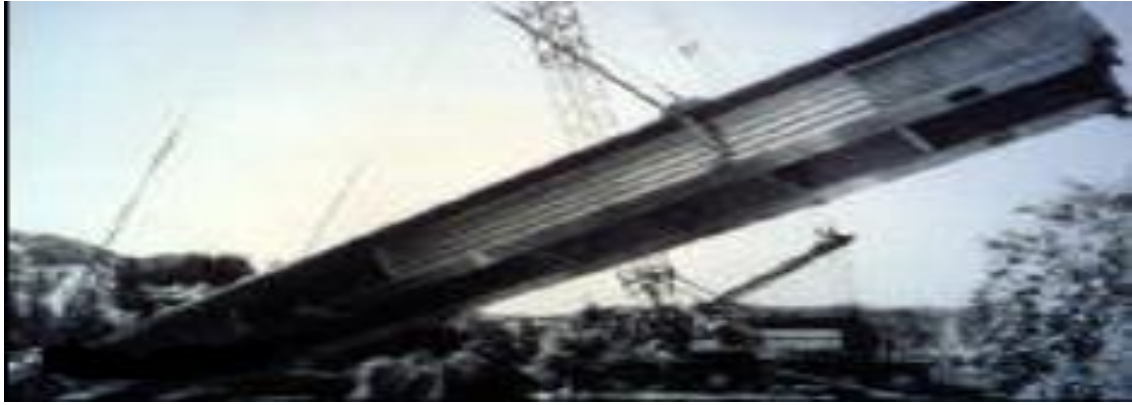
Figure1.6 The Foresmo Bridge in northern Norway is an example of the use of Al-Mg alloys for built up girders systems
