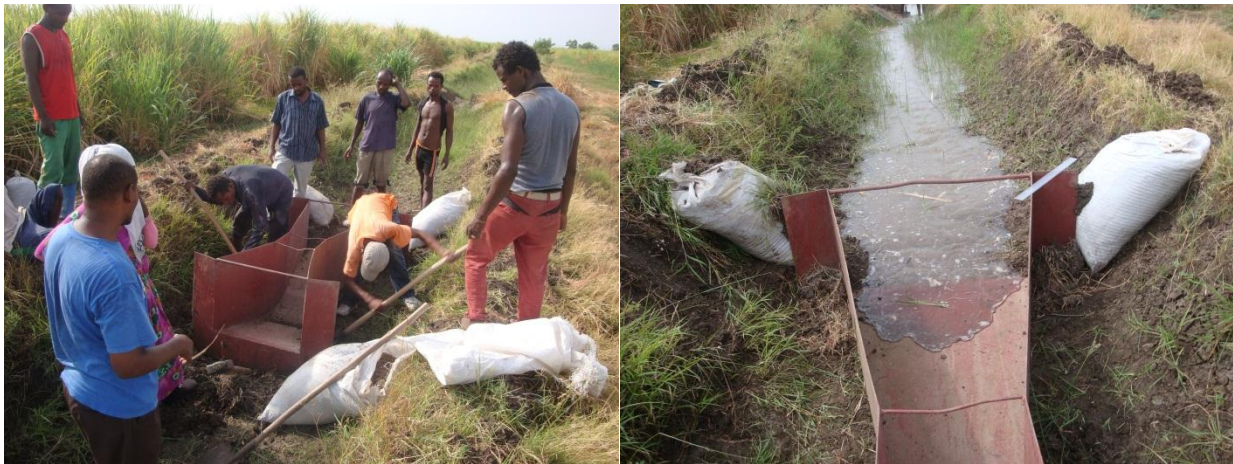
g) Setting up Parshall flumes for estimation of tertiary conveyance efficiency, Tendaho
