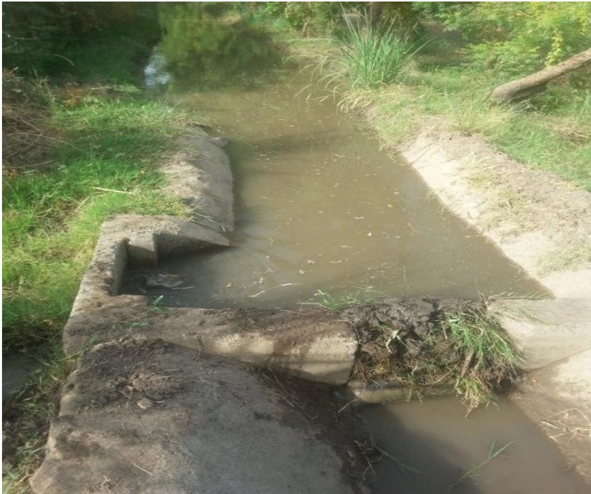
d) Tertiary off-takes closed by mud and mud filled in sack
