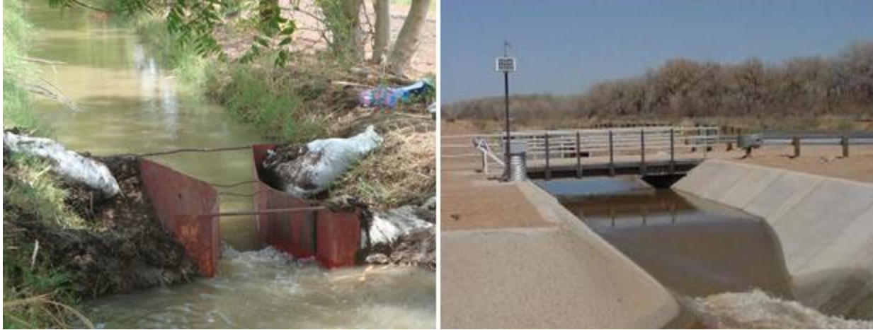
Plate 3 Typical flow measuring devices used in surface irrigation systems
