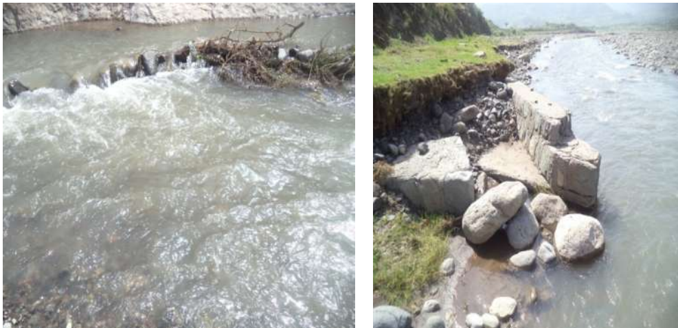
Figure 4.24 Traditional diversion structure and current condition of the designed intake structure
