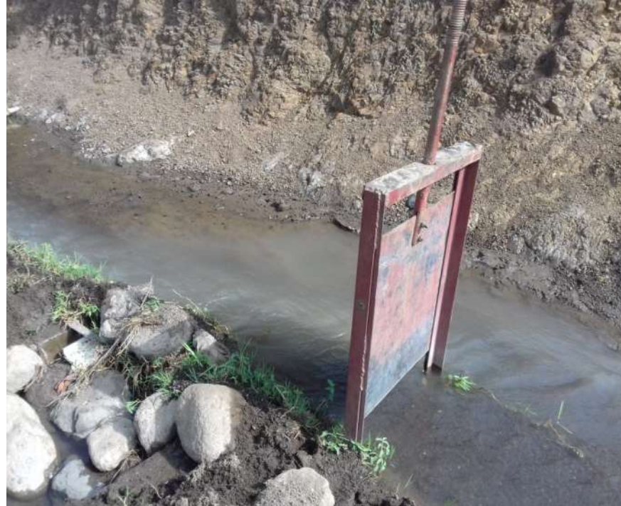
Appendix B-1 Installation of Current meter instrument and figure showing Malfunctioned flow regulator
