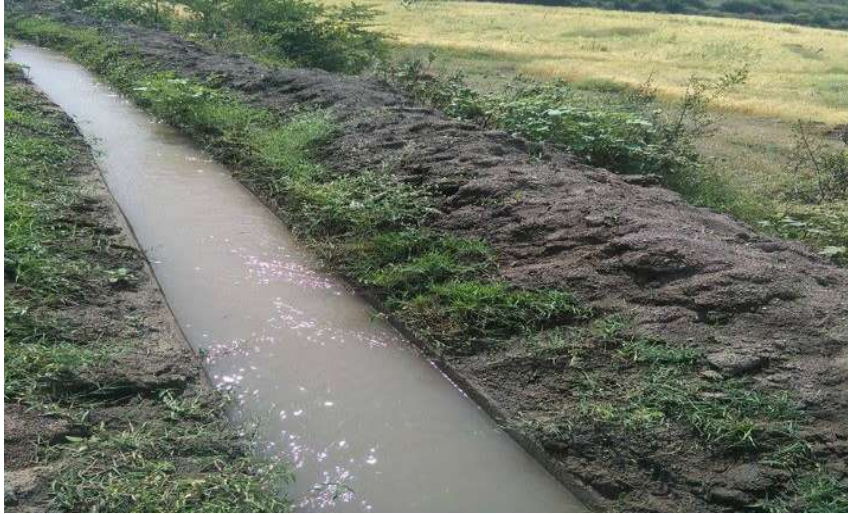
Figure 4.25 Remarkable improvement in canal sediment cleaning (October 2, 2017)
