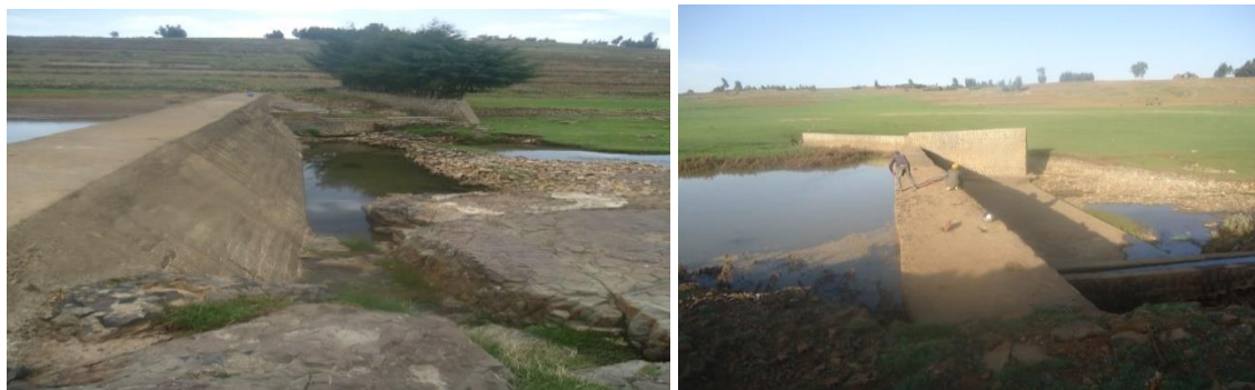
Figure 4.1 Kendbersha and Fiadiango_1 weirs constructed without under sluice and divide wall
